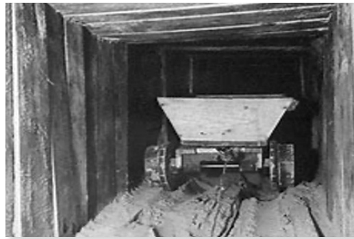
The tunnel measured 2 feet by 2 feet. The trolley was used to haul sand from the digging face. Note the rails. This was designed by Wally Floody.
